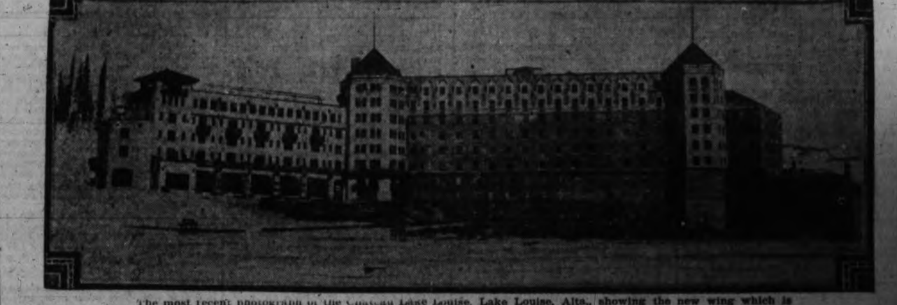
The most recent photograph of the Canadian Lake Louise, Lake Louise, Alta., showing the new wing which is practically completed. All interior work will be finished well in advance of June 15, the date set for the opening of the big mountain hotel for the summer season.
